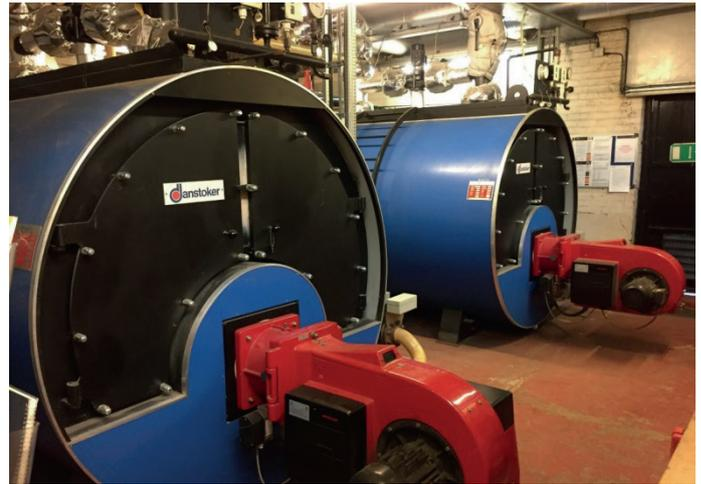
Figure 1.1 Image of the two 2MW gas-fired boilers within the Energy Centre.
